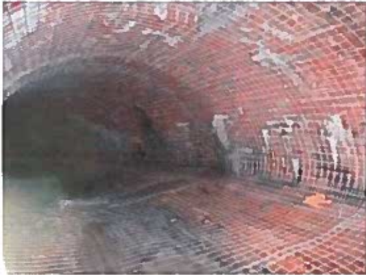
Mesh prior to Gunite lining
