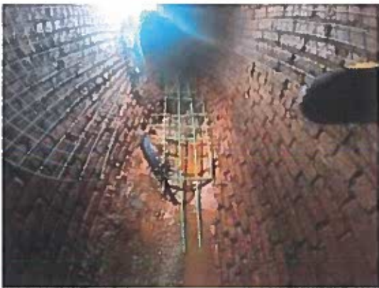
4 th District Brick Sewer Invert Repair
