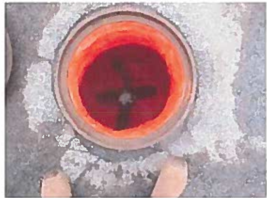
Manhole Rehab Lining
