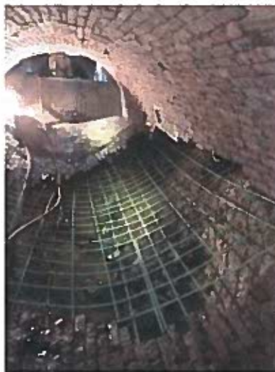
2 nd District Brick Sewer Repair
