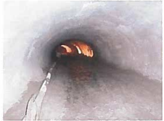
Finished Gunite Lining
